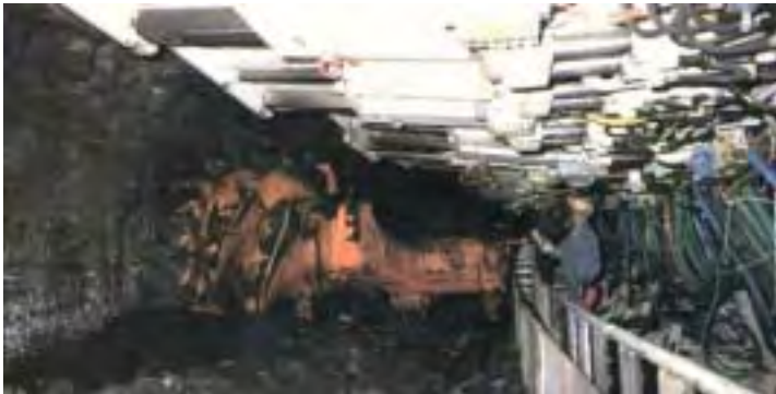
Longwall mining (SD Mining) drum shearer and shield support
